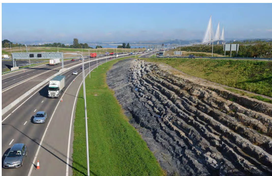
Beds of sandstone and shale exposed in new road cuttings that border the M90 on its approach to the recently completed Queensferry Crossing over the Forth. Photo by Lorne Gill/SNH
