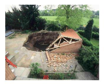
New suffosion sinkholes are nearly all formed by rainstorms, new drainage inputs or water table decline; they are therefore largely avoidable if the gospel of drainage control is obeyed.
