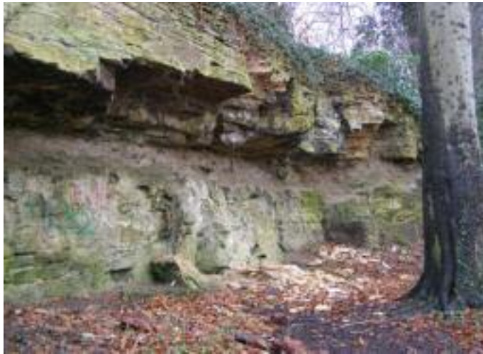
Permian limestones beside the River Wharfe at Boston Spa
