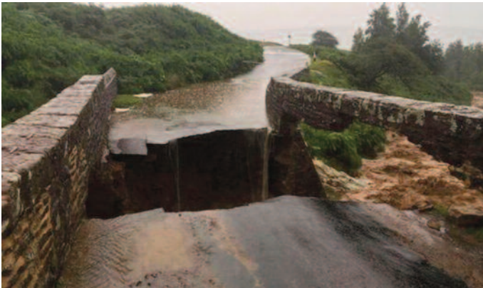
This bridge, near Grinton in the Yorkshire Dales, was washed away
