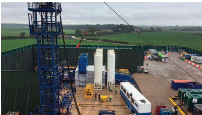
A view of the Preston New Road site, taken just a few days before the latest 2.9 earthquake (Image: Sky News)
