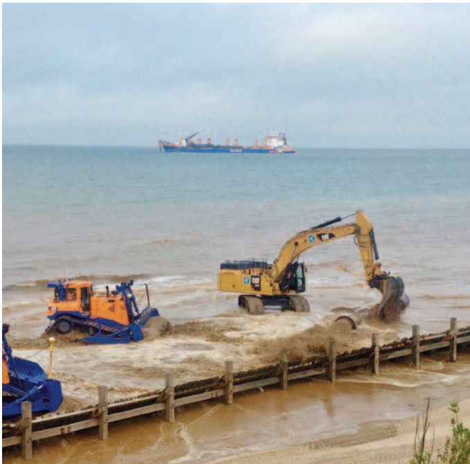
At work on the beach at Bacton in early July, with the dredger in the background. (Image: Twitter)
