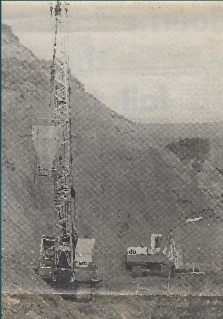
Coastal protection work November 1983.
