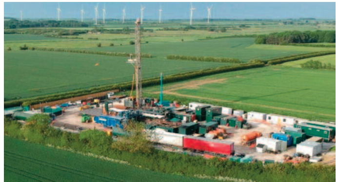
The drilling site near to the village of West Newton in Holderness (Image: Raebald Resources)
