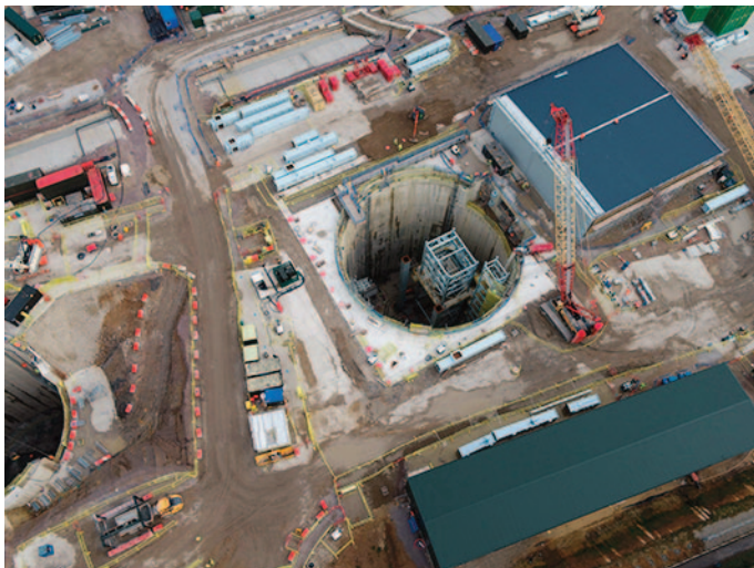
The Woodsmith Mine construction site south of Whitby. (Image: International Construction/Anglo American)
